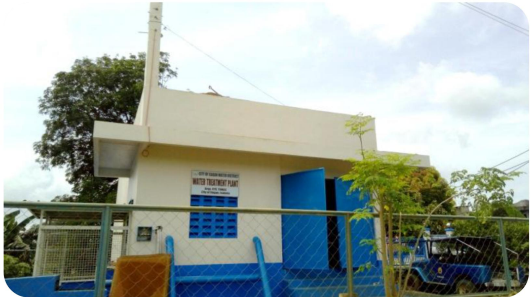
STO. TOMAS WATER TREATMENT PLANT
