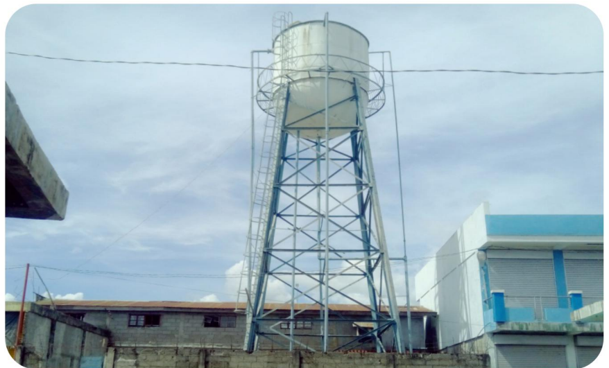
BALIGATAN ELEMENTARY SCHOOL PUMPING STATION
