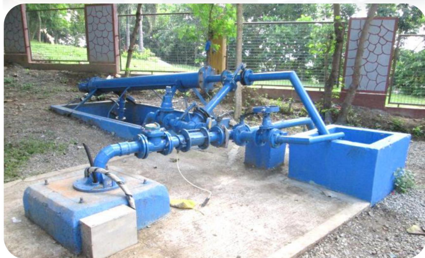
SINGLE STAGE ON LINE SAND FILTER MEDIA ILAGAN SOUTH CENTRAL SCHOOL PUMPING STATION
